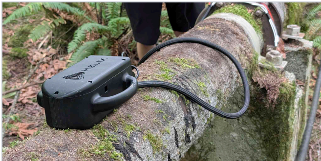
HELIX PEC screening on an in-service line — no insulation removal.
