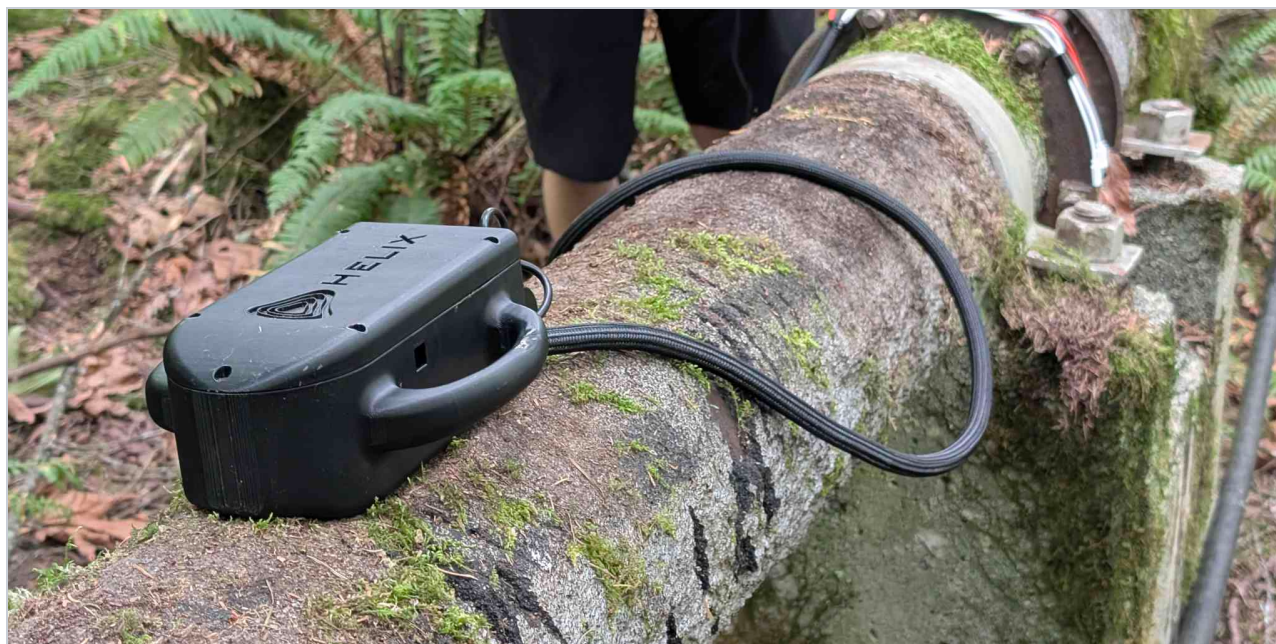
The HELIX PEC scanner on an in-service line — screening proceeds from the outside, through the coating.
